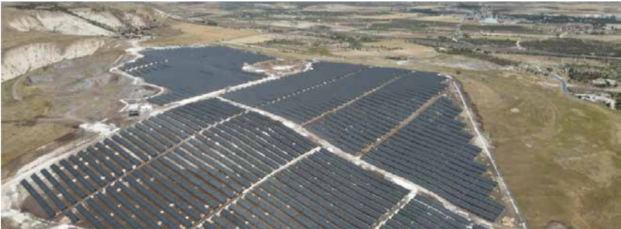
18MW PV Plant, Turkey
